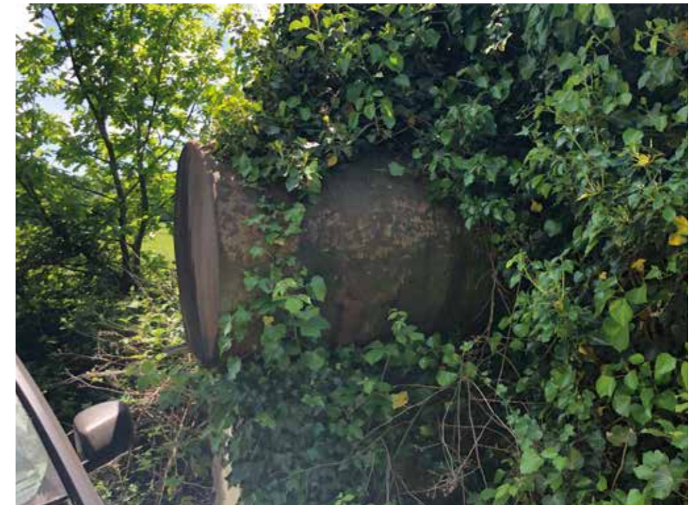
18. Redundant above ground storage tank at Sleepbrook Farm
